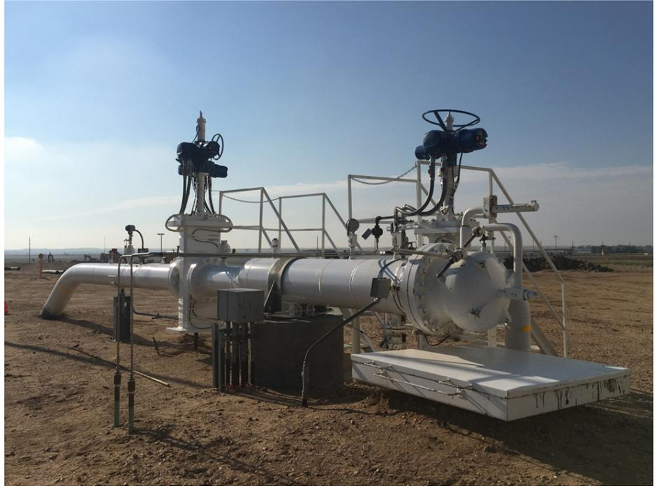
Top photo shows the pig receiver. Bottom panel shows interior of receiver after pigging run before treatment program (left) and after initiation of FORSA PAO2016 paraffin dispersant prior to each pig run (right).
