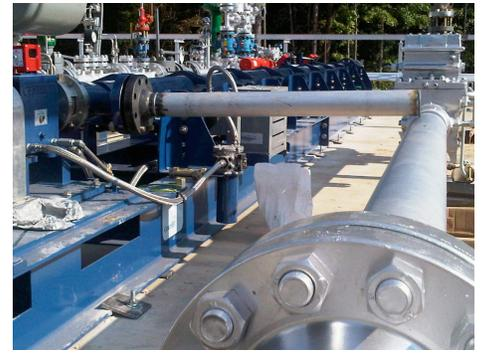
BHGE CO<sub>2</sub> HPump surface pumping system permanent installation.
