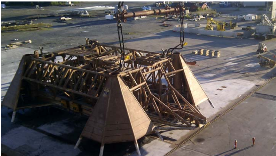
Subsea template (note scale compared to personnel on the ground at lower right).
