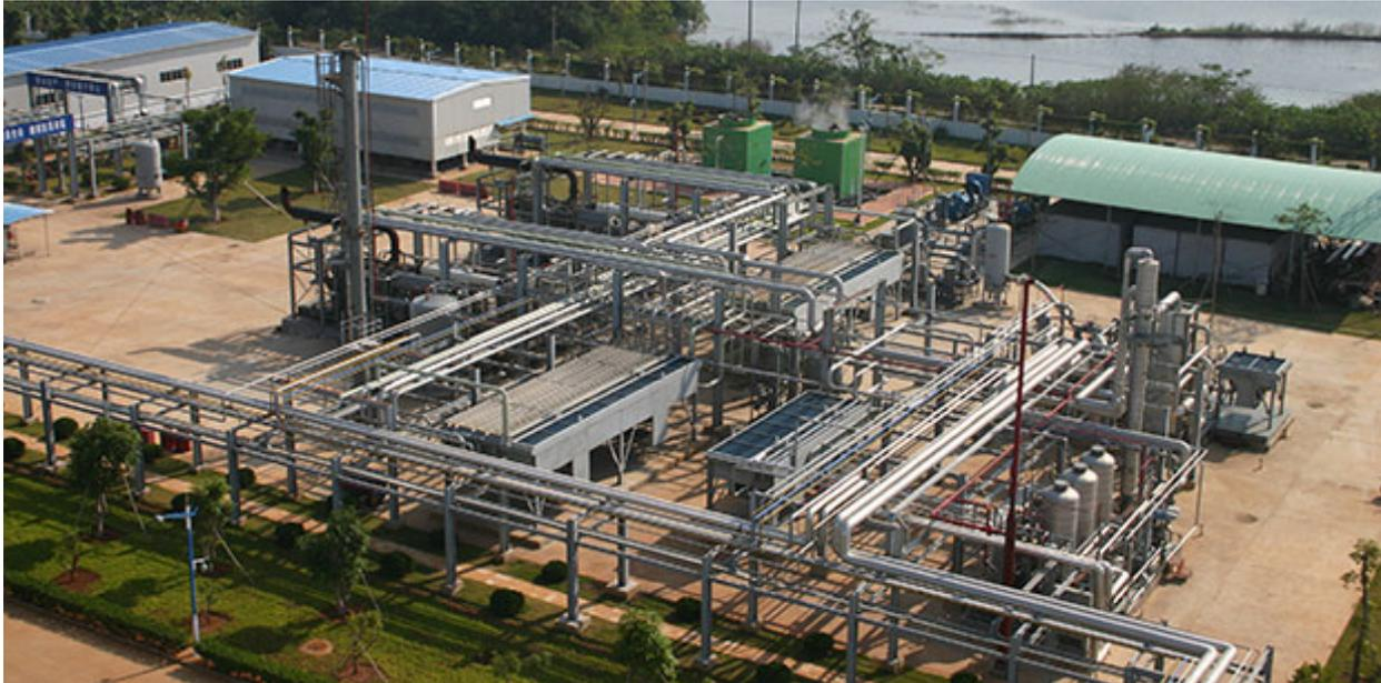
120,000 GPD, CH<sub>4</sub> refrigeration cycle LNG plant
