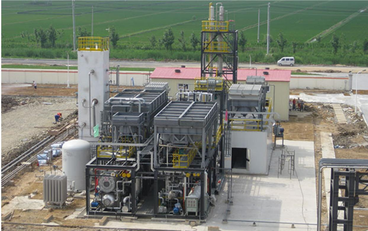
25,000 - 50,000 pre-cooled mixed refrigerant cycle LNG plant
