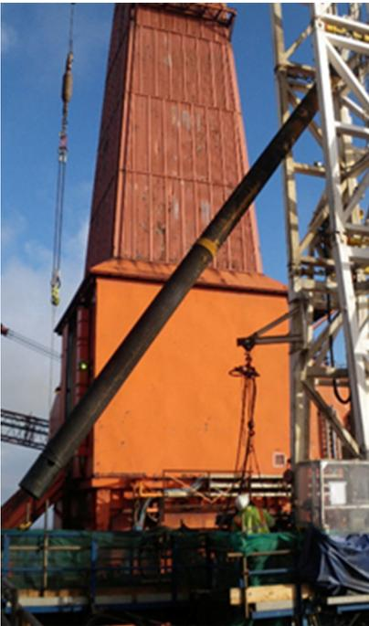
The Mastiff RIS performed casing and conductor recovery on 23 platform wells prior to removal of the topside platform module.
